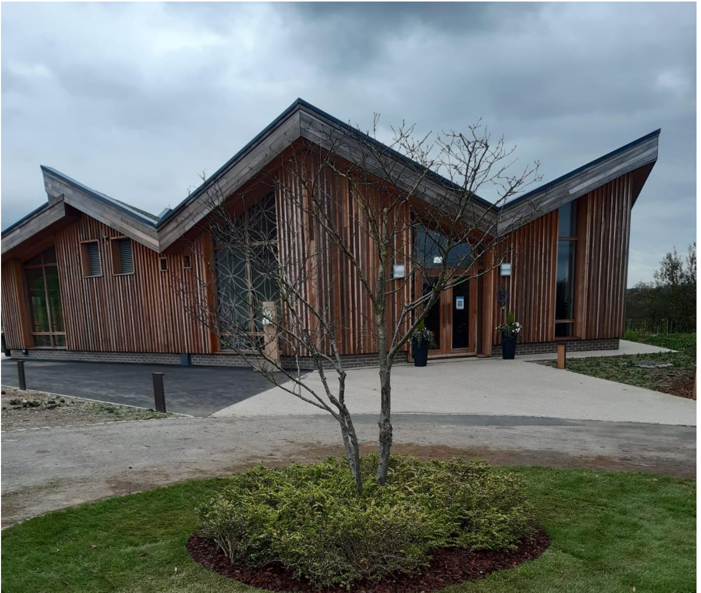
Woodland Hall and offices
